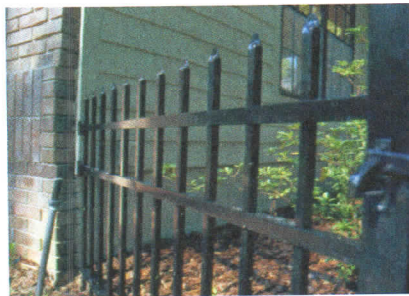
Use non-flammable fencing if attached to the house such as metal.
