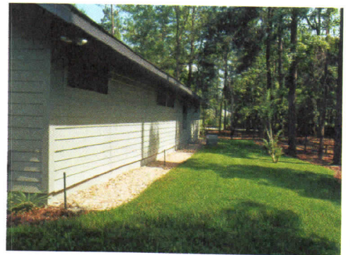
Use pebbles instead of mulch near the home's foundation where possible.
